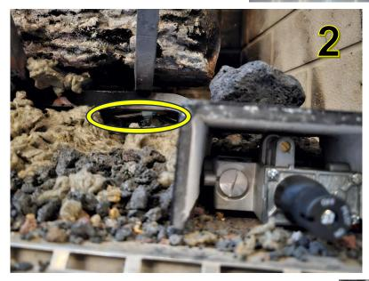
Visually locate the Pilot, which can be found underneath the right side of the logs.
