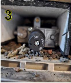
\*\*Should the Pilot go out, the safety switch automatically turns off the flow of gas. Simply turn to "OFF" and restart the lighting process to re-light the fireplace.
